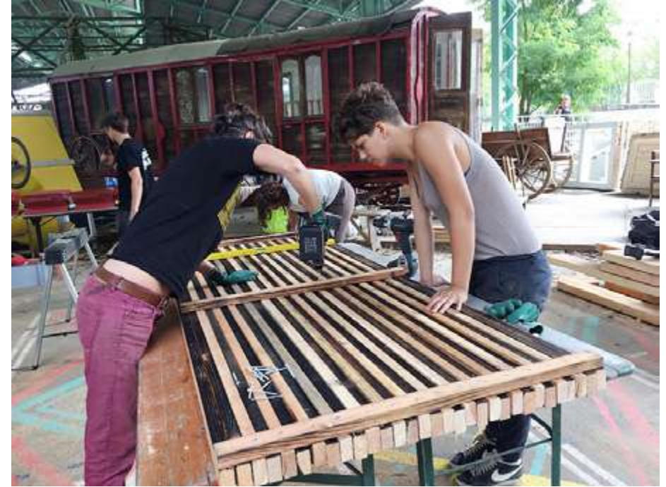
screwing to get the external cladding
