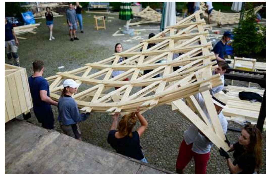
moving the structure
