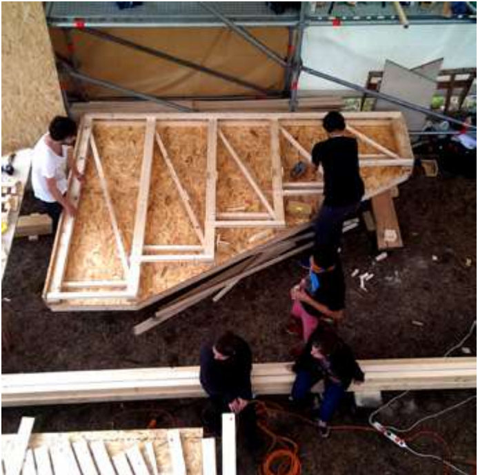
building the frame with the jig
