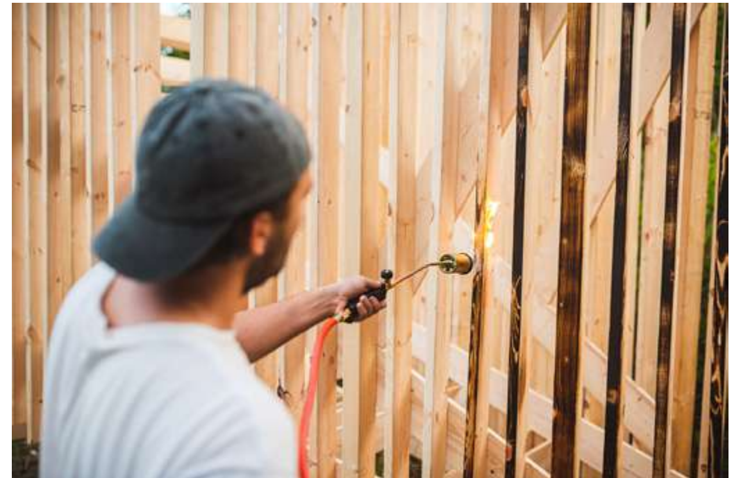
finishing and protecting the wood by burning it
