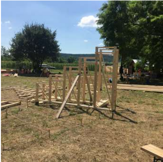
placing the frames on site
