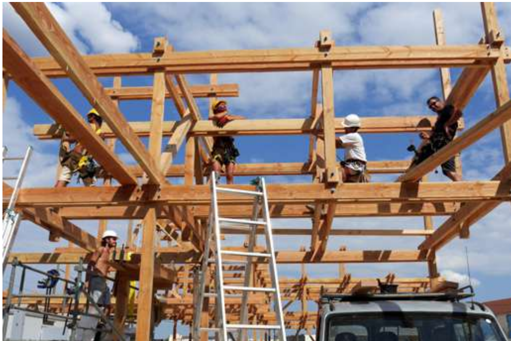
building the grid structure
