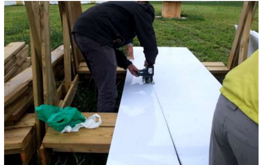
cutting the polycarbonate jig with a circular saw
