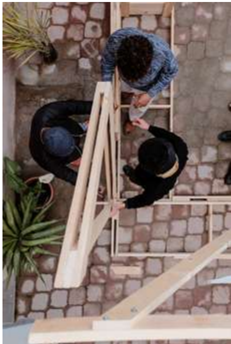
placing a frame on the platform
