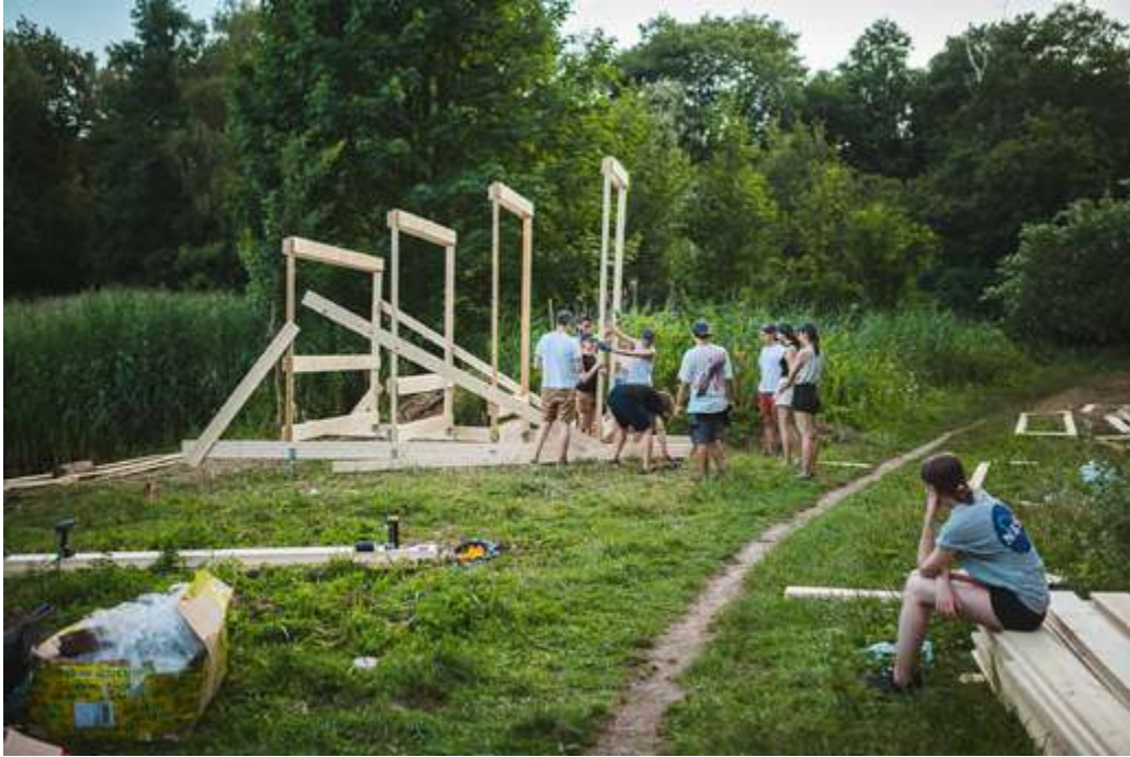
placing the vertical frames
