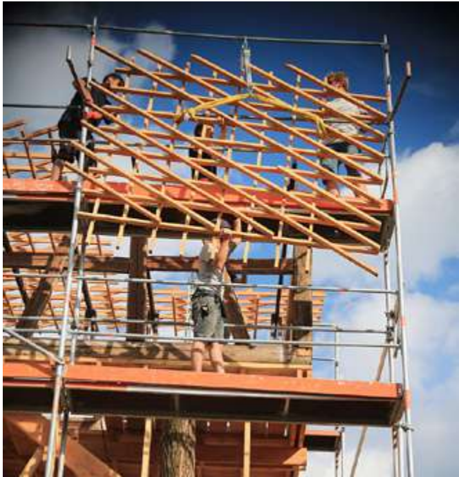
raising the roof structure with a pulley
