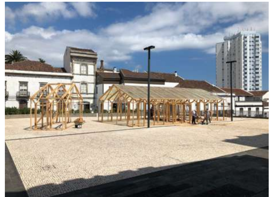
overall view of the construction in progress
