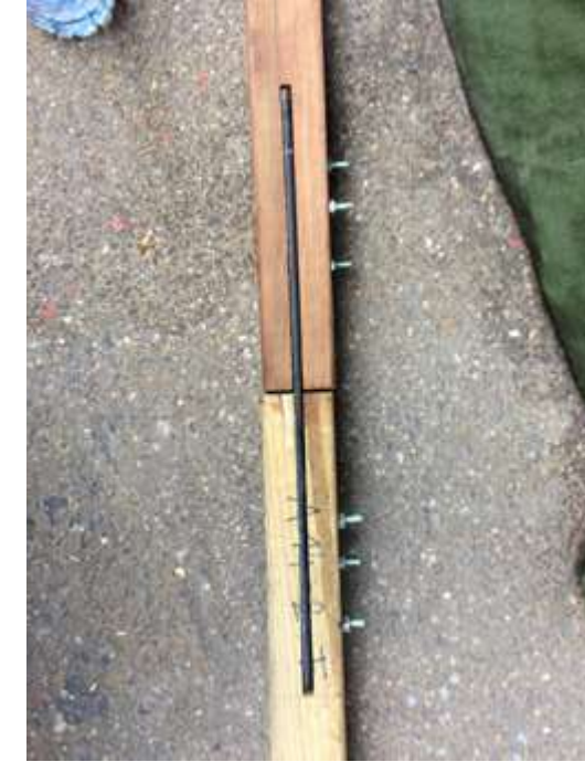
joining the wood with a metallic plate
