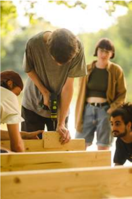
drilling with a jig
