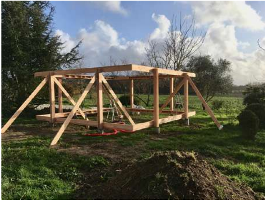
stabilizing the outer frame
