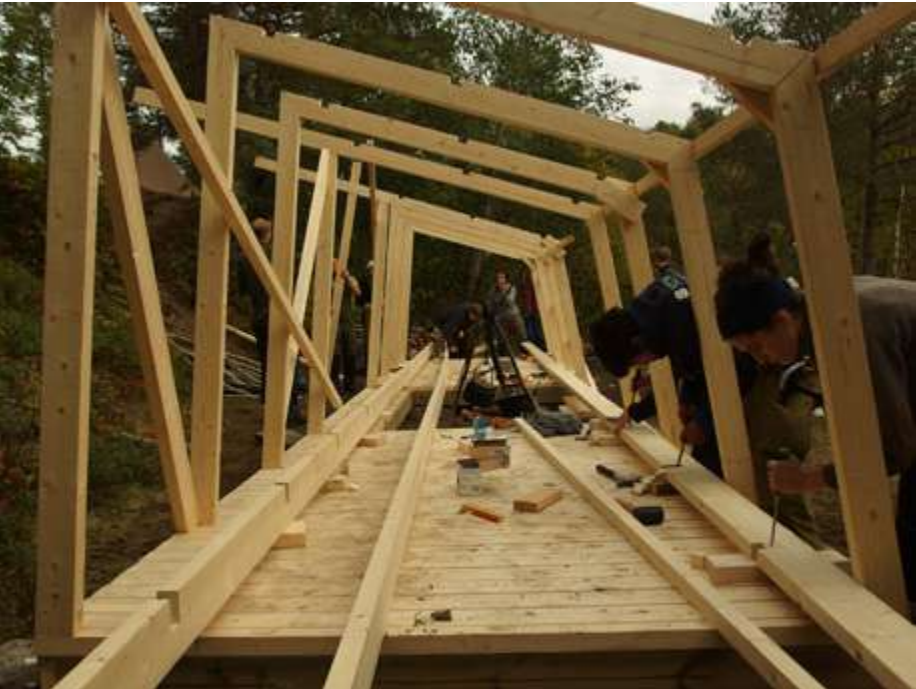
cutting the horizontal beam with chisels
