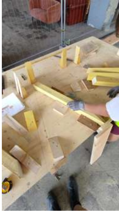
jig to accelerate the building process
