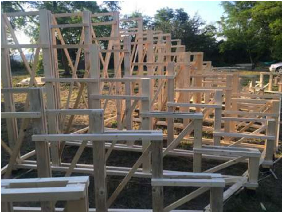
optimising the frame production thanks to jigs
