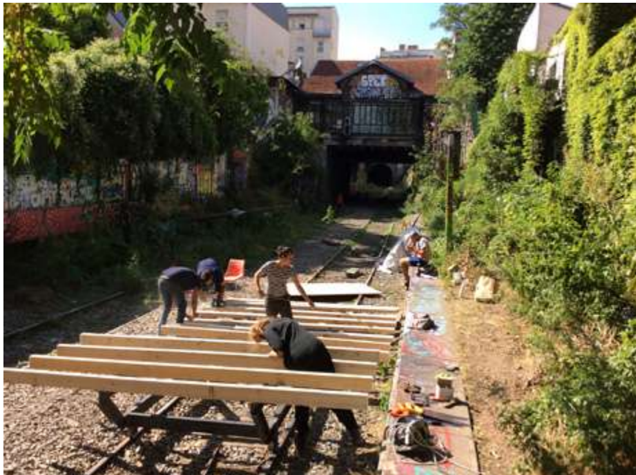
assembling the horizontal beams on the moving load-bearing frame
