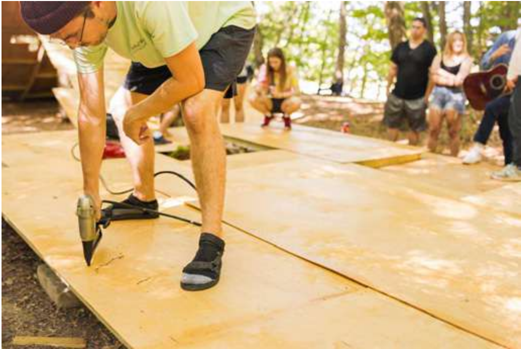
nailing with a pneumatic tool
