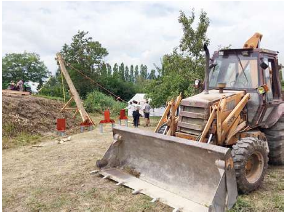
lifting the post
