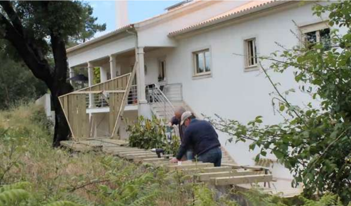
building the frist frame
