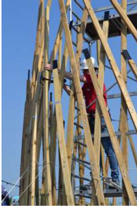
clamping and drilling
