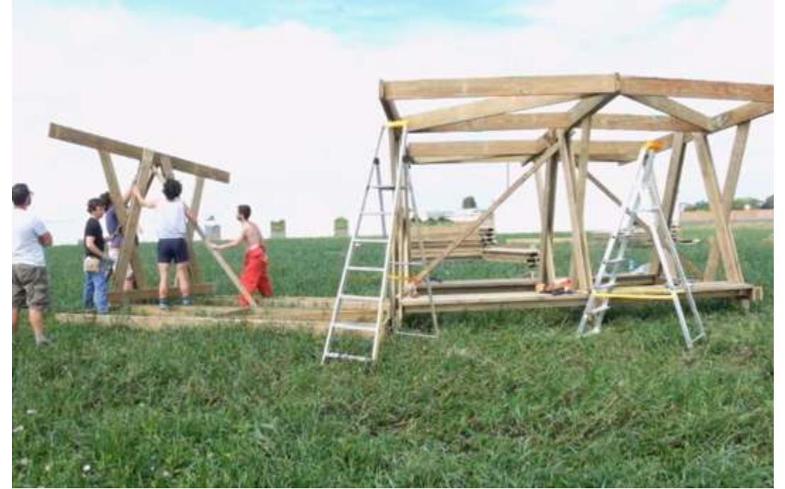
stabilizing the structure
