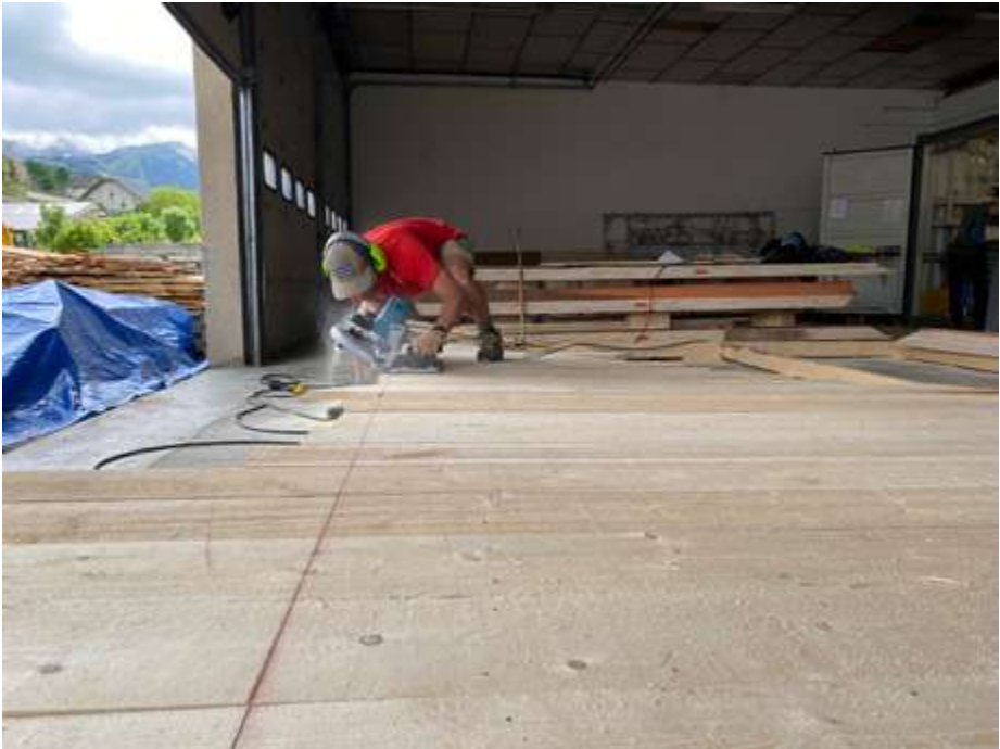
cutting the lumber to make the inner structure
