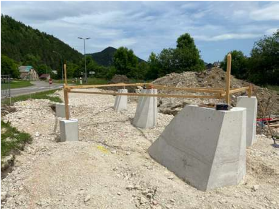
installing the concrete foundations
