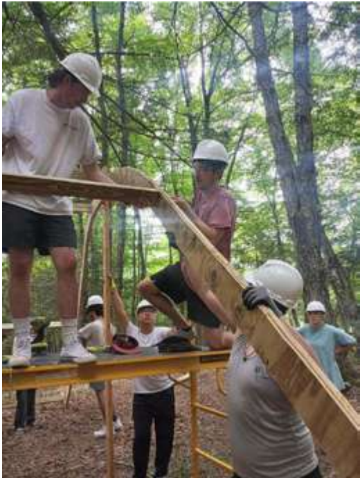
team work positioning the laminated archs
