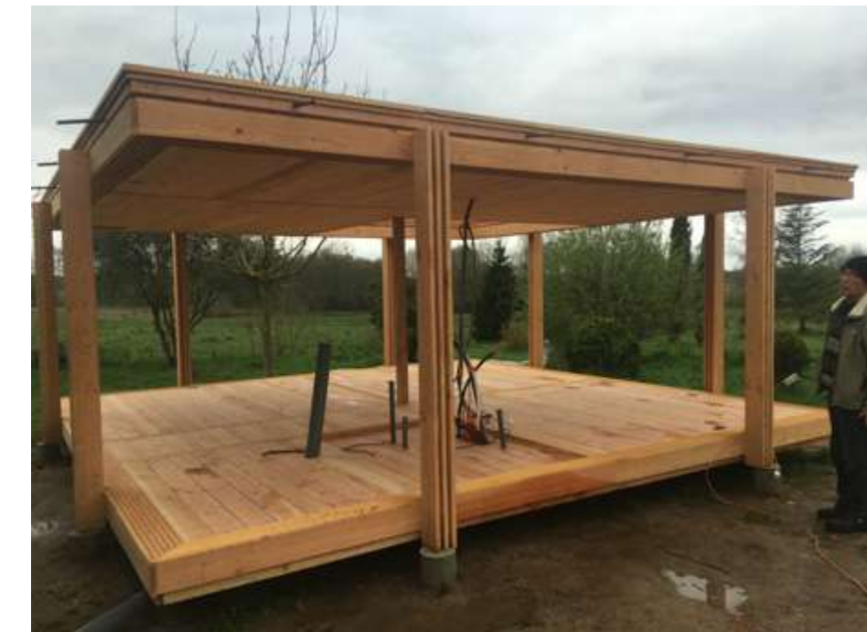
decking and covering
