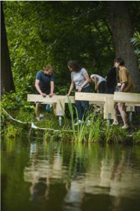
assembling the structure
