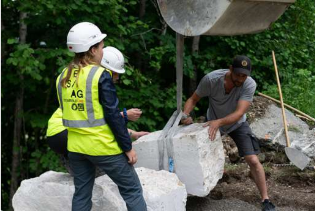
placing the boulder foundations
