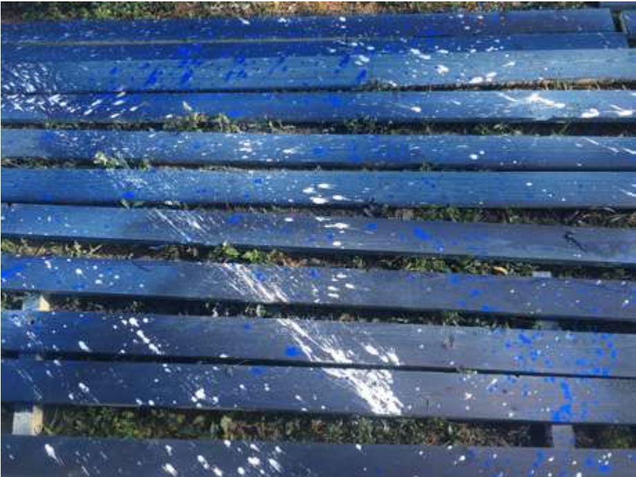
detailed view of the finishing
