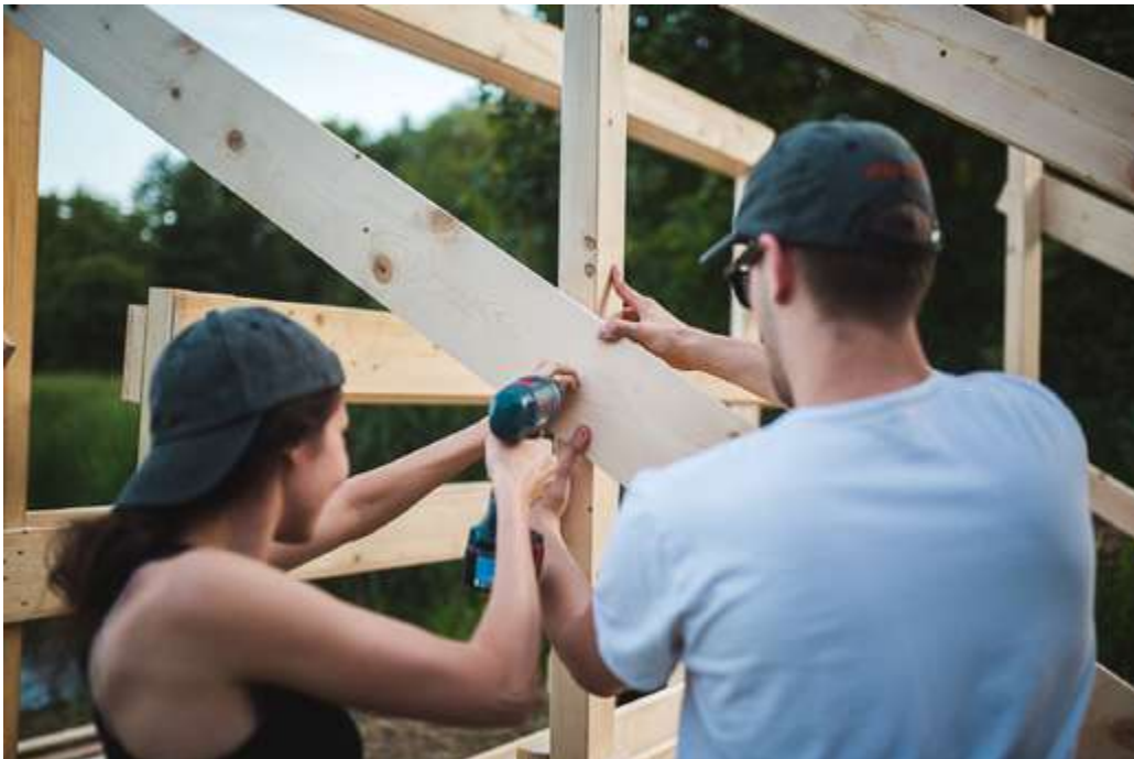
bracing the structure with diagonal planks
