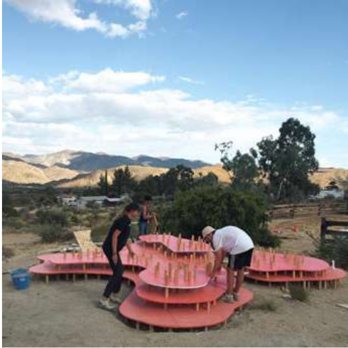
adjusting the plywood decks
