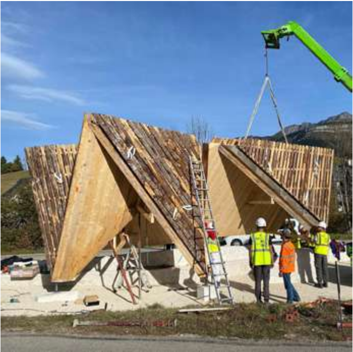
lifting the structure
