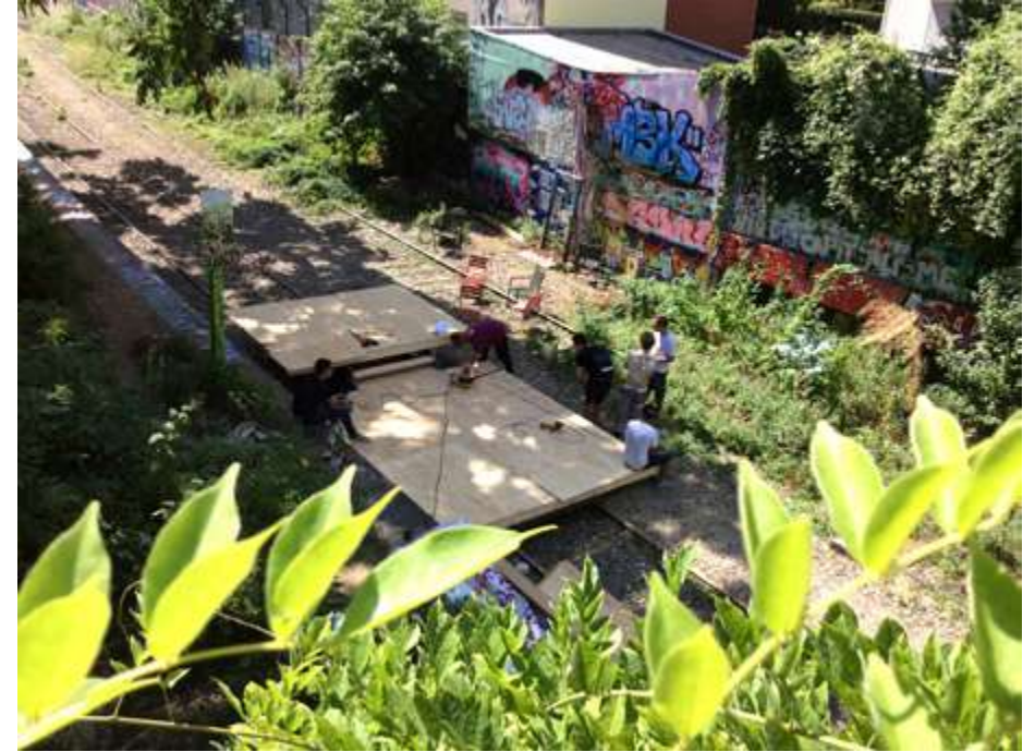
decking the mobile structure
