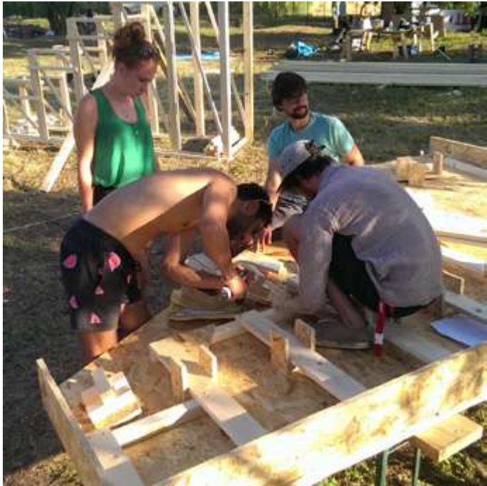
assembling using a jig
