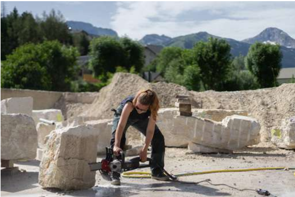
cutting the boulder foundations
