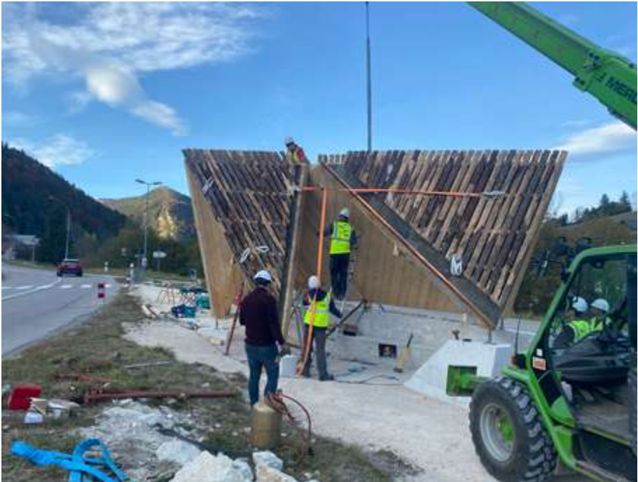
placing the structures
