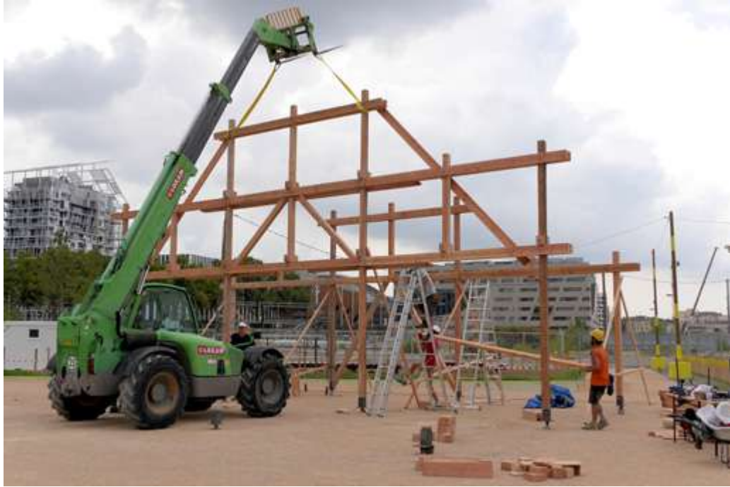
raising the frame with a forklift
