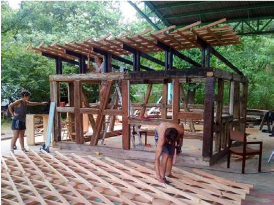
building the roof structure
