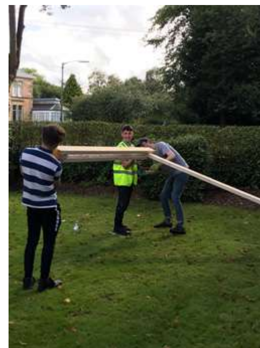
lifting the frame
