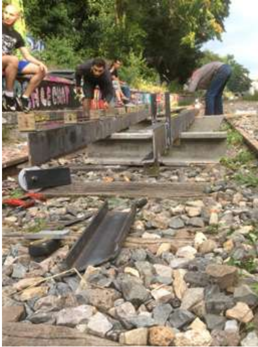
building the metallic frame
