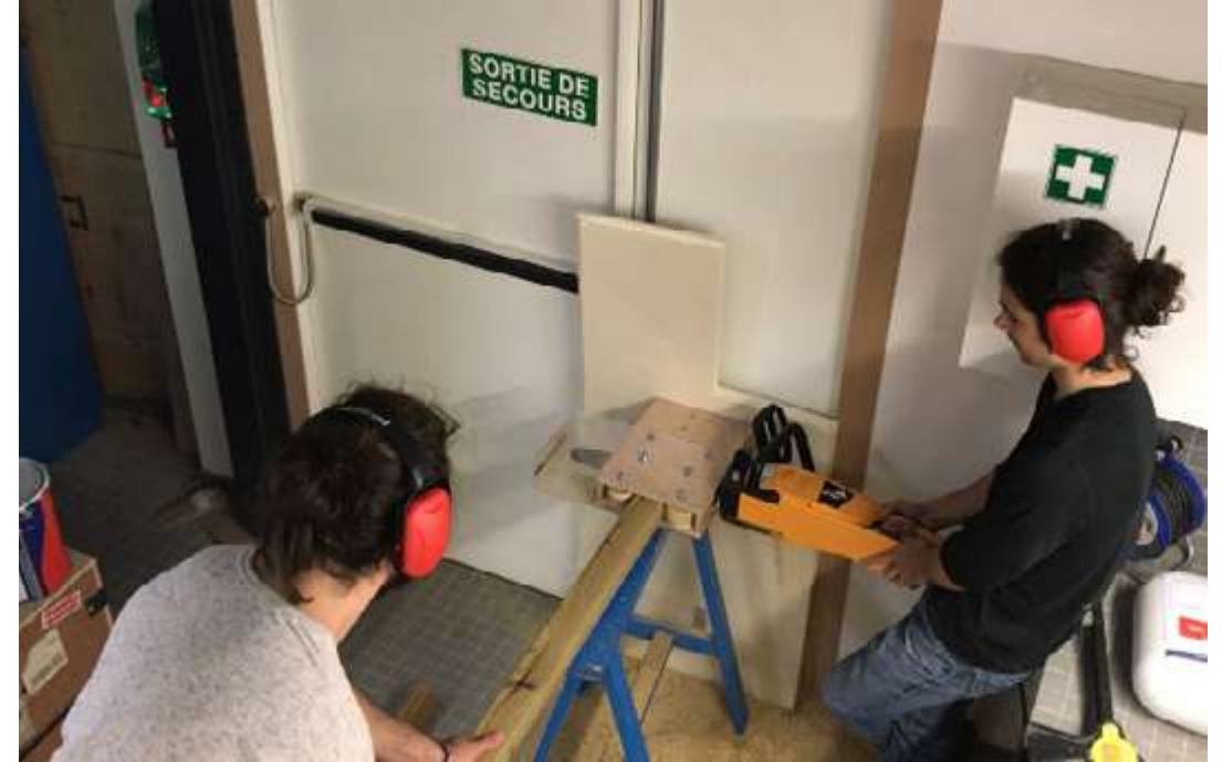
cutting grooves in the wood with a chainsaw
