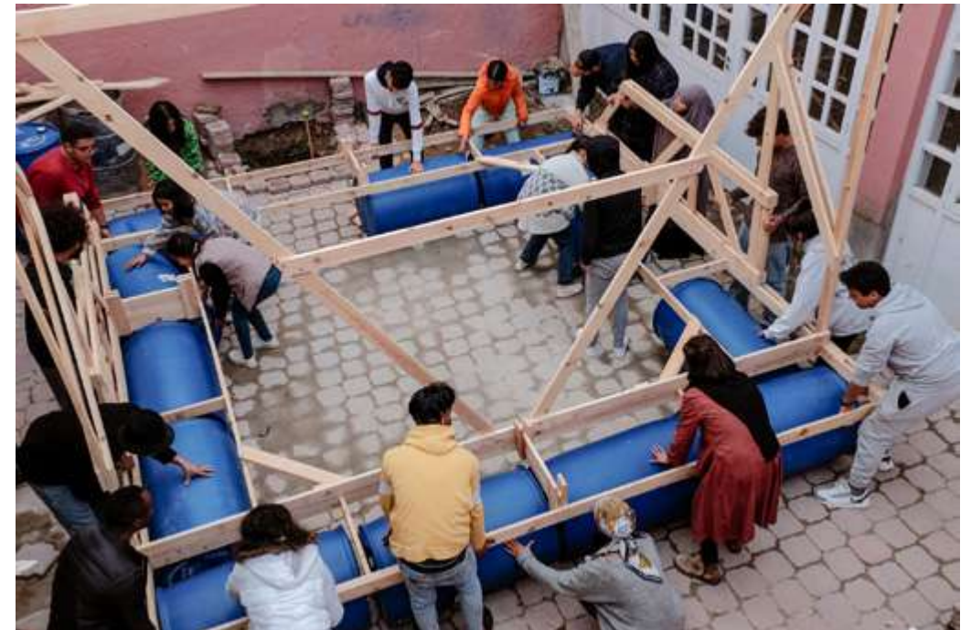
lifting the structure all together on the blue barrels
