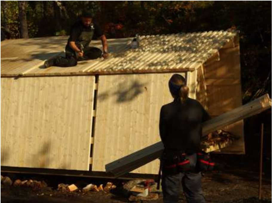
covering the roof
