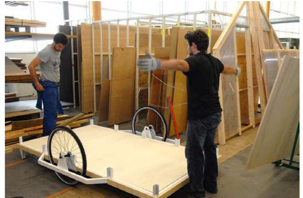
build the load-bearing frame
