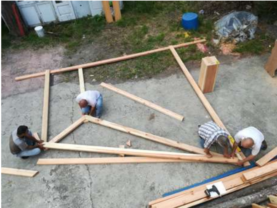
building the frames
