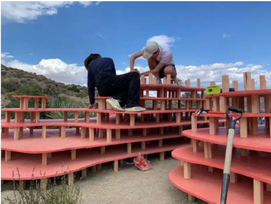
screwing the plywood decks
