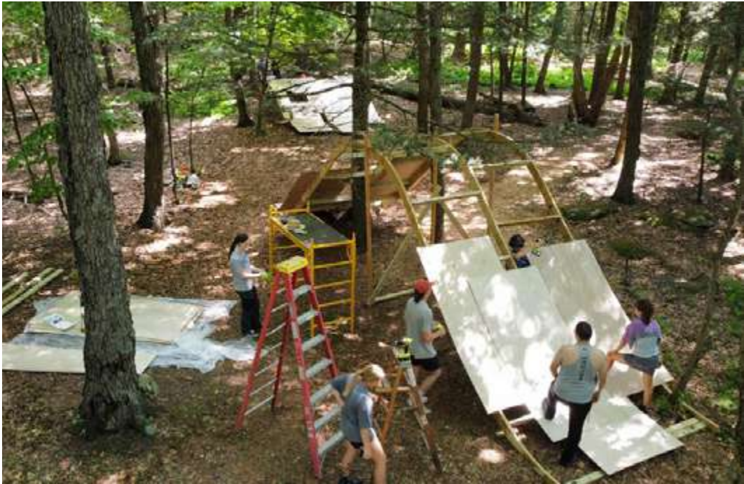
fixing the decks on the structure
