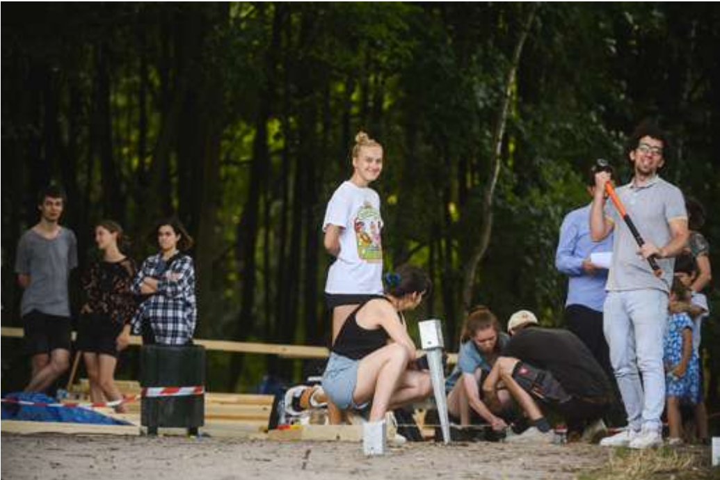
placing the foundations
