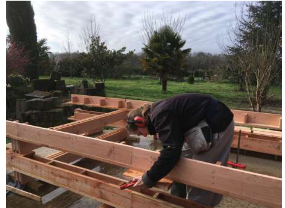
building the structure
