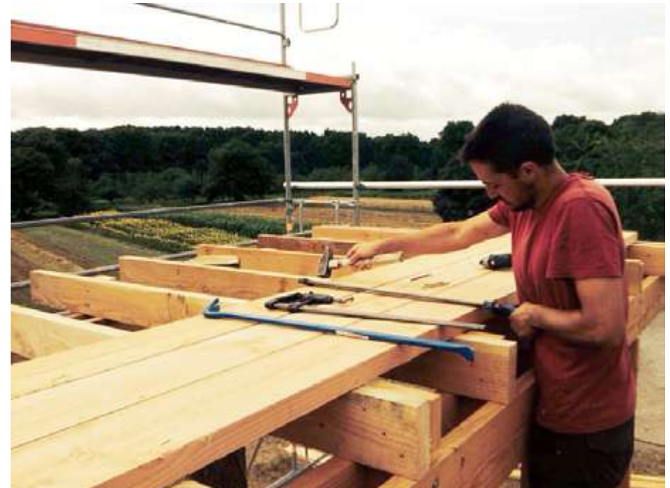
clamping the planks
