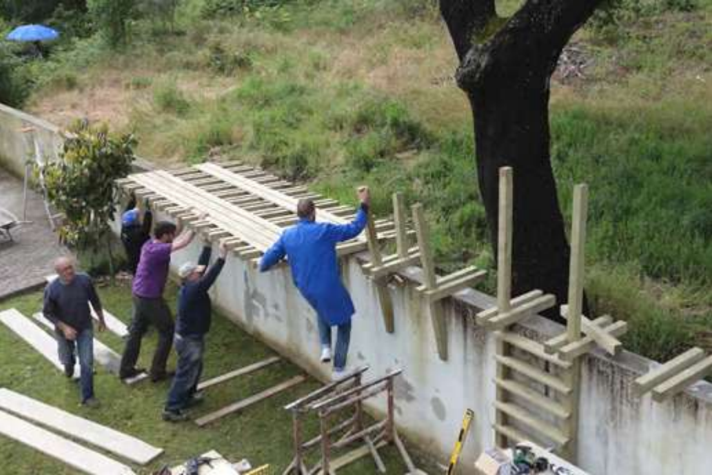
building the platform
