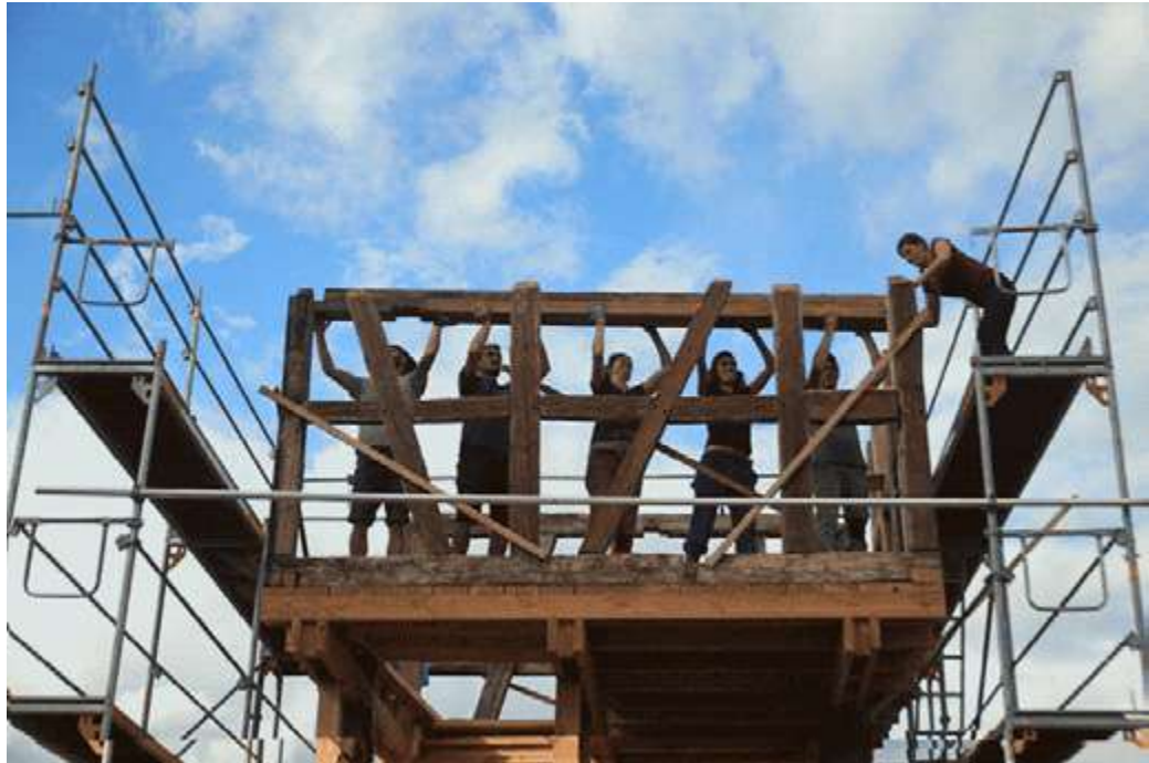
lifting the beam all together
