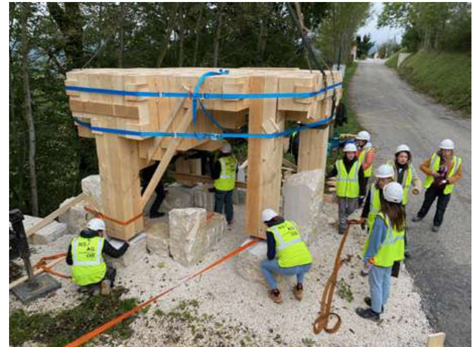
placing the structure on the foundations
