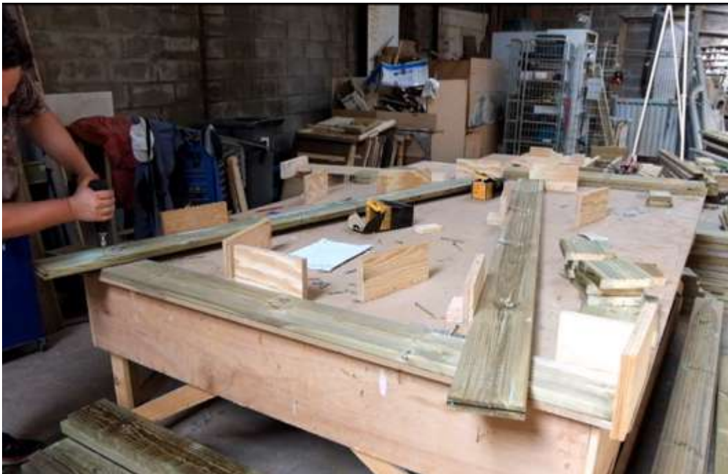
building the frames with jigs
