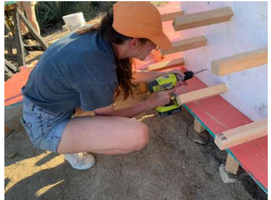
screwing the wooden pegs
