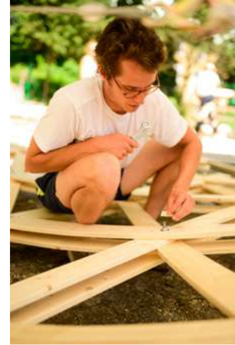
threaded rods and nuts assembly
