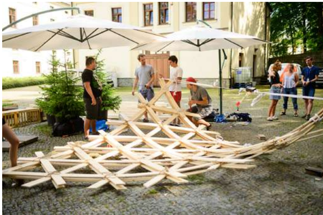
bending the wood with a ratchet belt
