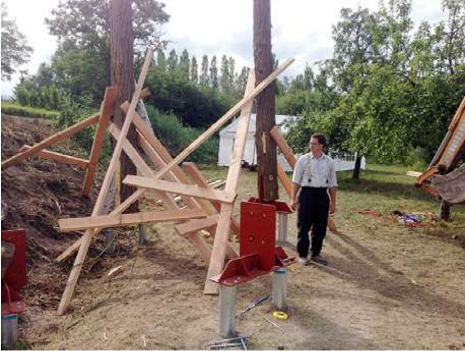
bracing the posts on their foundations for stability
