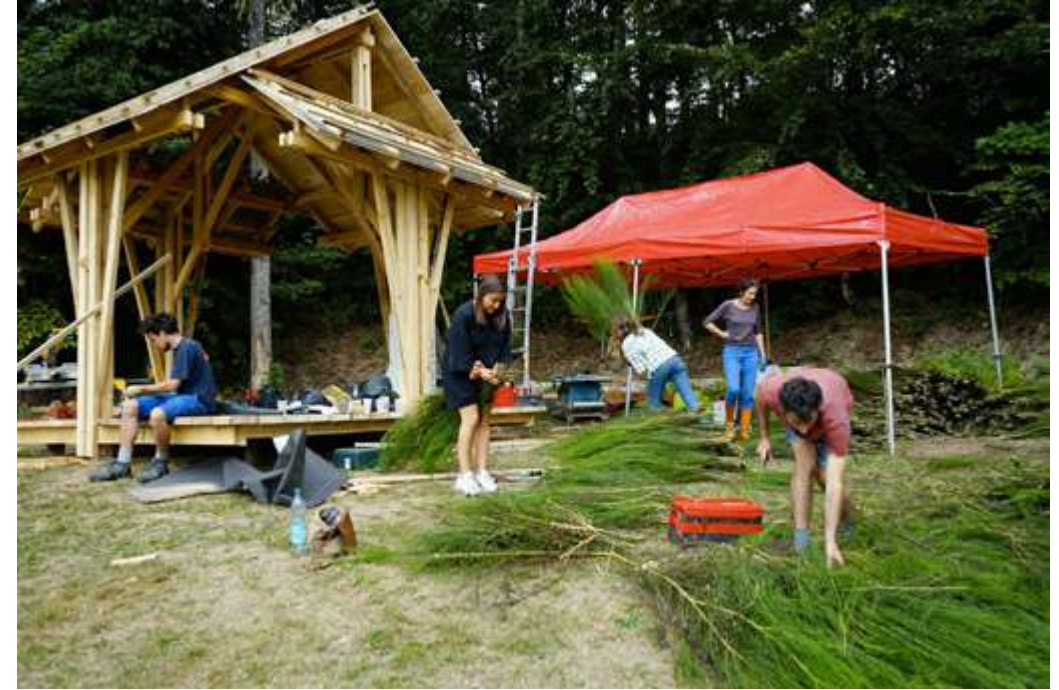
preparing the roof covering with tree leaves
