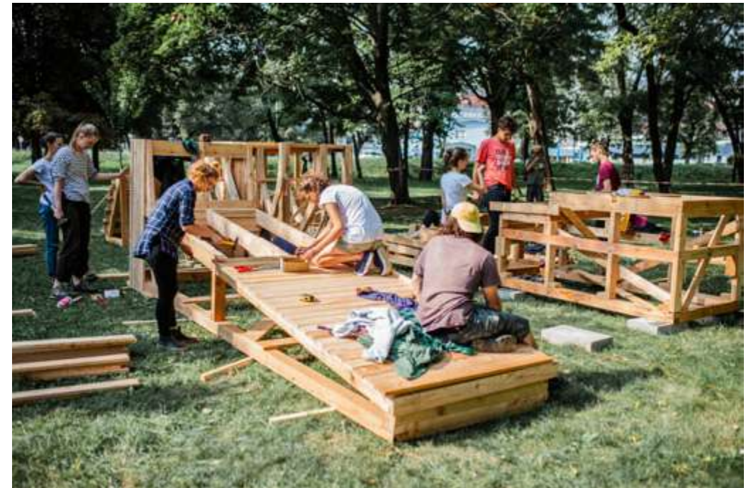
decking the structure
